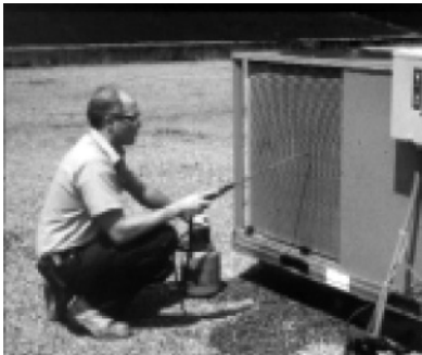
Fig. 1 - Applying Coil Cleaner
