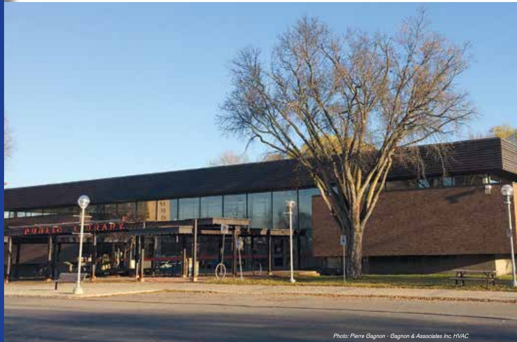
Photo: Pierre Gagnon - Gagnon & Associates Inc. HVAC
